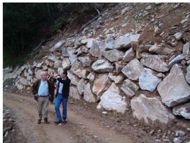
Fig. 9. Anrocamente la debleu Anrockments at cut
